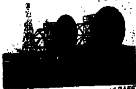
Wardlaw Hill, part of the military-owned RAFFTS transmission system.
